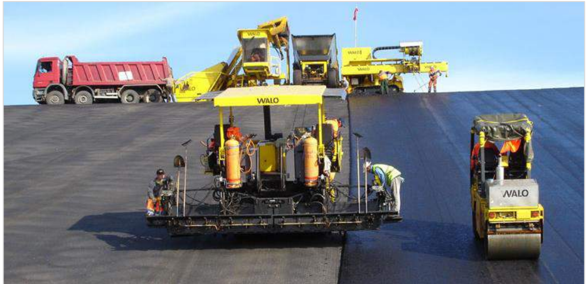
Figure 45 - Illustration of asphalt paver on dam face
