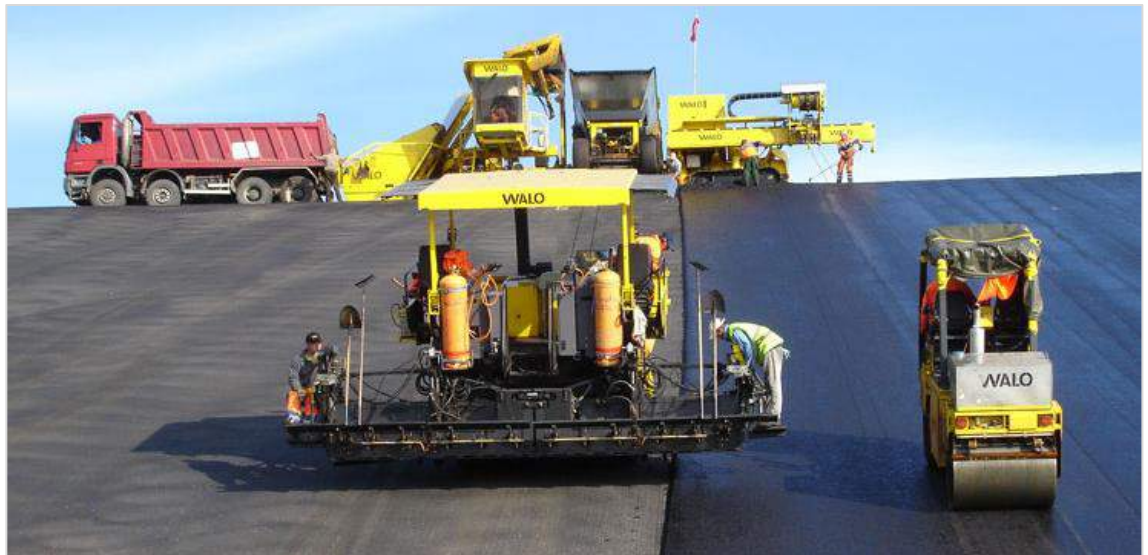
Figure 47 - Illustration of asphalt paver on dam face
