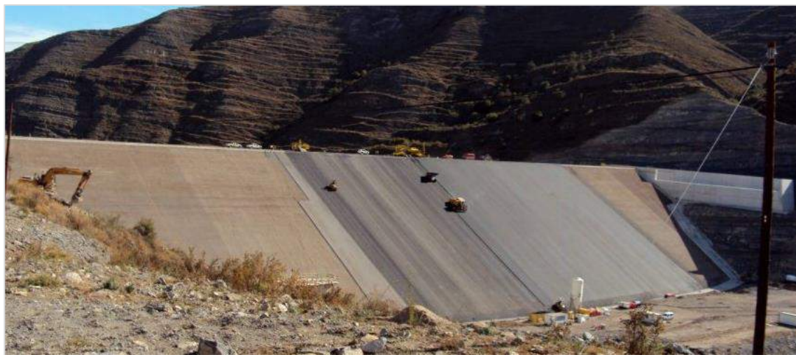
Figure 46 - Illustration of upstream face asphalt lining (Terroba dam - Walo)
